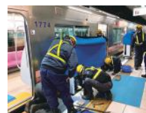
From delivery to installation
