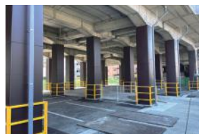
Elevated bridge anti-earthquake strengthening work
