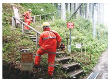
Undergrowth clearing work
