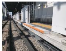
Installation of rubber bumpers for fall prevention Platform elevation
