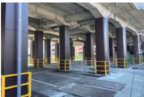
Elevated bridge anti-earthquake strengthening work
