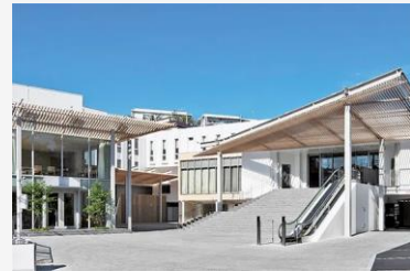
Repair work to YOKOHAMA SEIEN designed and supervised by the world-renowned architect Kengo Kuma
