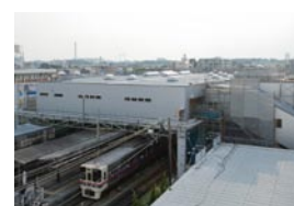
Construction work on the new elevated station building at Sakurajosui Station
