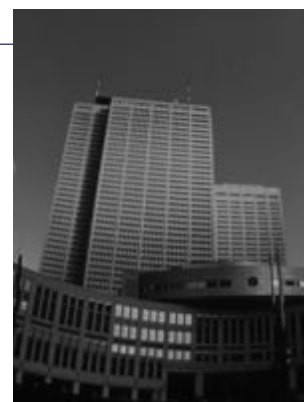
The Company’s flagship Keio Plaza Hotel
