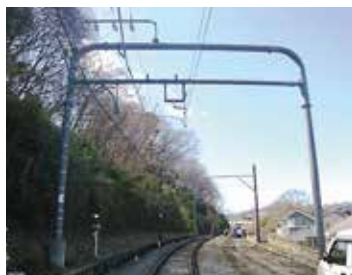
(更新後)鋼管柱
