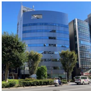
Nomura Fudosan Higashi Nihonbashi Building (plan to acquire in FY2022)
