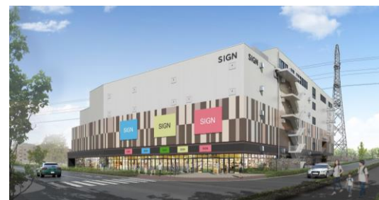
Development plan for front of Tamasakai Station (Completion planned for winter FY2023)
