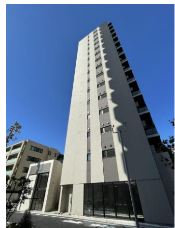
MODIER KOMAZAWA (Completed in June 2023)
