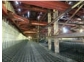
Below the Kokuryo Station Tracks
