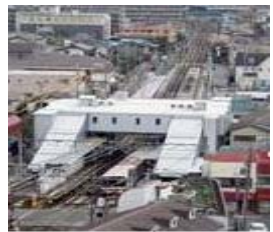
Structure prior to switch to underground station
