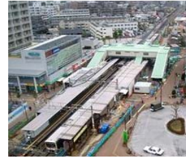
Structure prior to switch to underground station
