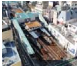
Structure prior to switch to underground station
