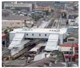
Structure prior to switch to underground station
