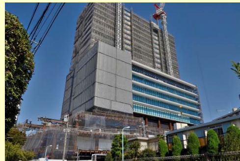
New construction site
