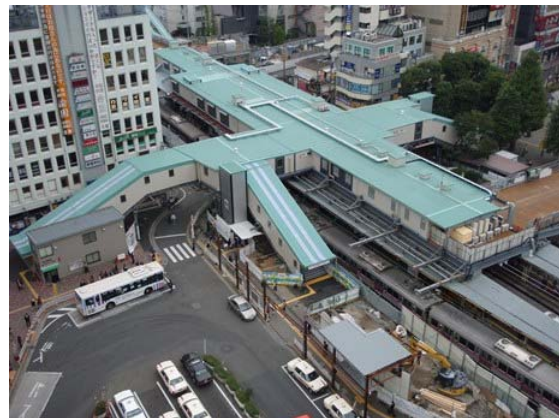
Structure prior to switch to underground station
