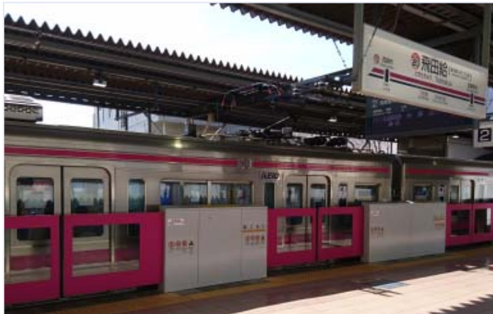
These sliding platform doors went into service on platform 2 of Tobitakyu Station in March 2019
