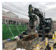
Construction around Meidaimae Station
