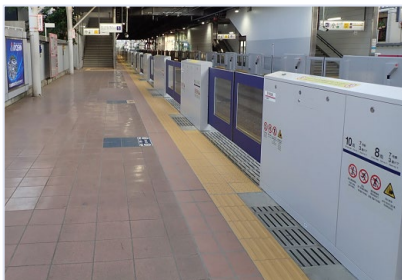
Installation of platform doors (Tobitakyu Station)
