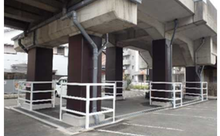
《Work to strengthen resilience of elevated sections to earthquakes》
