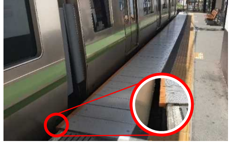
《Installation of rubber bumpers for fall prevention》
