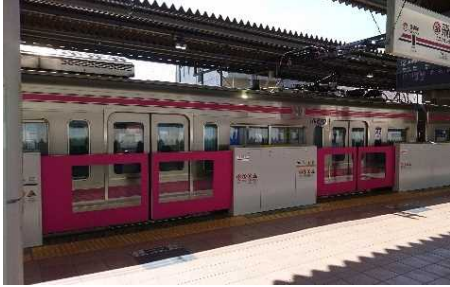
《Installation of platform doors》
