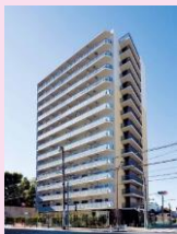
ACOLT Nakano Fujimicho (Completed January 2023)
