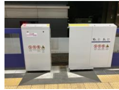
New style of platform door
