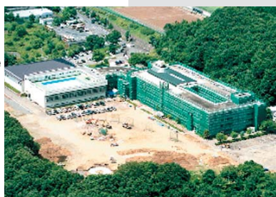
Takaonomori Wakuwaku Village ( Under construction )
