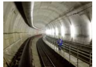
Tunnel Excavation between Kokuryo Station and Chofu Station
