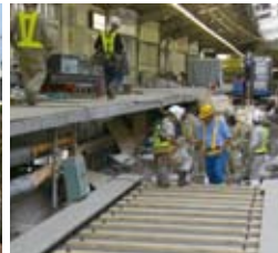
Construction at Kichijoji Station
