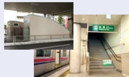
The newly constructed evacuation passageway at the Hatagaya Station (bottom) and above-ground exit (top)
