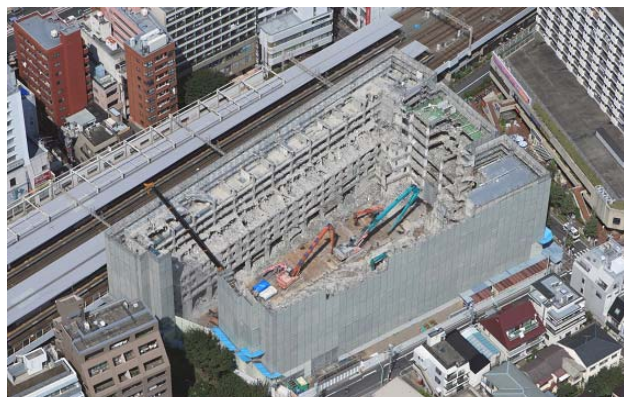
Keio Juuki Building during demolition work
