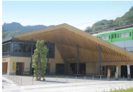
Renovation of Takaosanguchi Station
