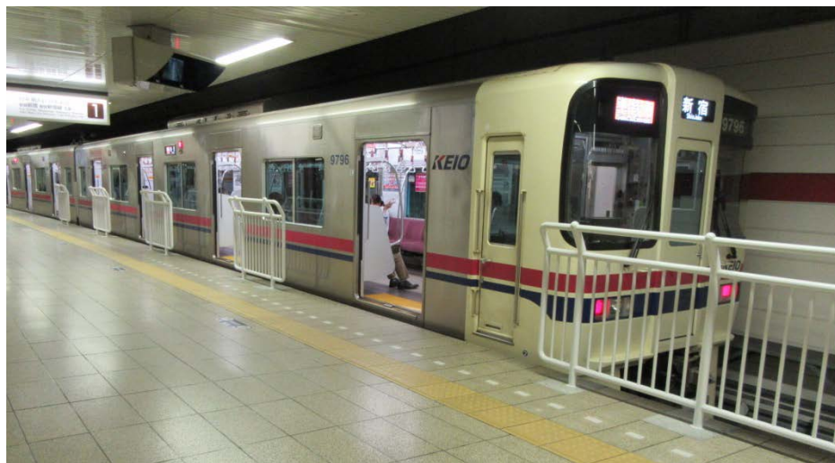
Example of fall prevention fencing (Keio-hachioji Station)
