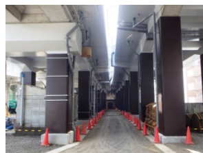
An elevated section following anti-earthquake strengthening
