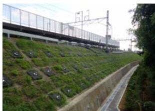
An embankment section following anti-earthquake strengthening
