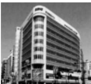
The Keio Shinjuku Oiwake Building, completed in April 2001
