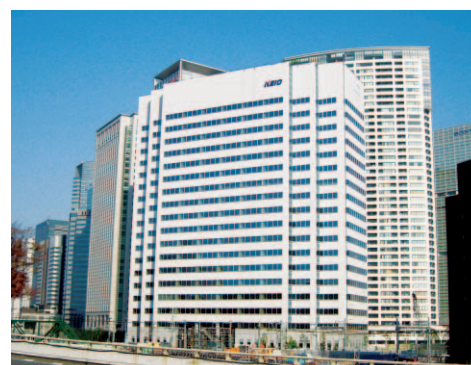
Keio Shinagawa Building
